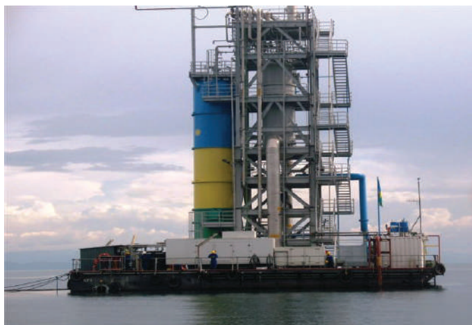
Fig 19.2: Methane power plant on Lake Kivu
