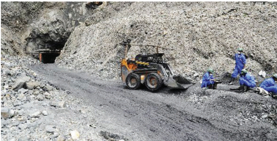
Fig 12.2: A mining process in Rulindo District, Northern Province
