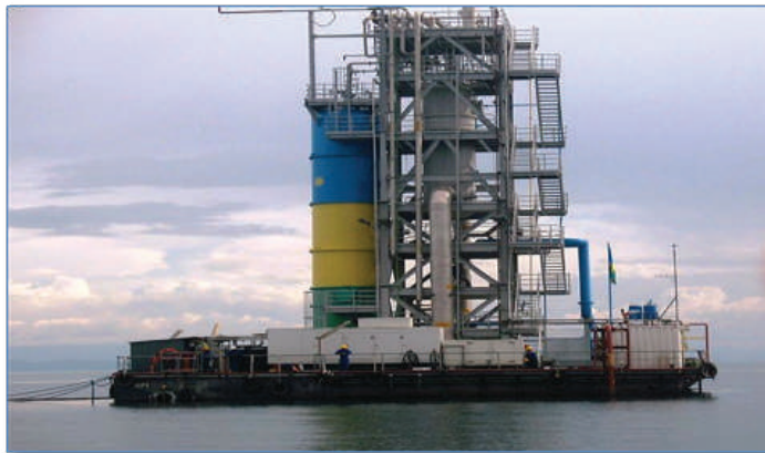
Fig 18.4: Extraction platform floating on Lake Kivu
